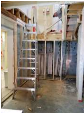
Wheel chair lift cut out from the lower level, looking up.
