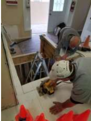
Wheel chair lift cut out, looking down from above.
